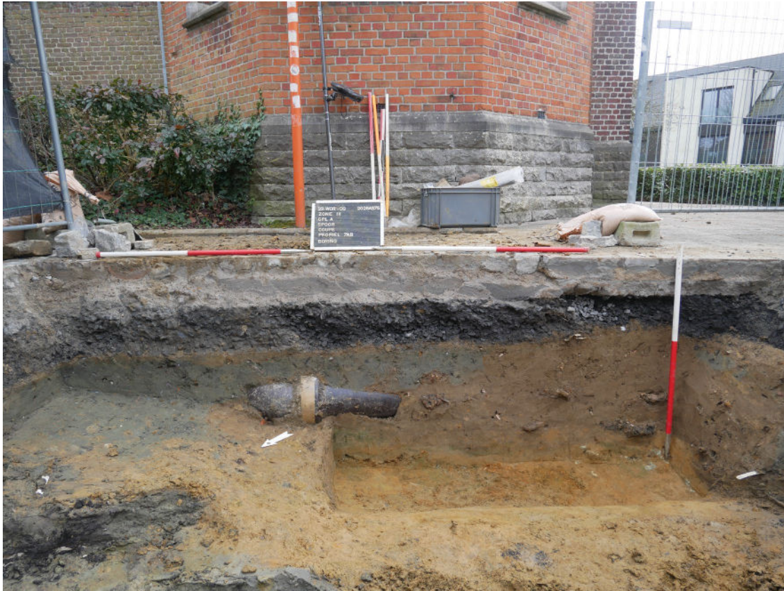
Foto 15: Profiel 7AB in zone III.
